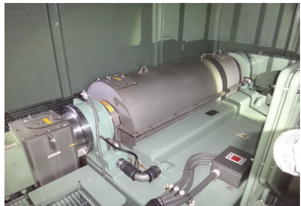
No. 2 汚泥濃縮機更新
