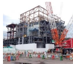
Installing a large cover for Unit 1
