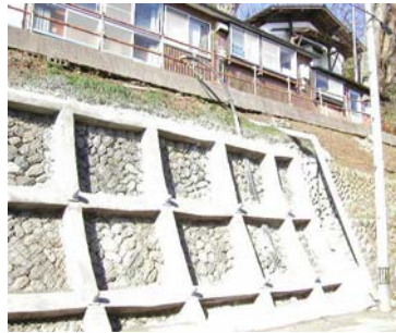
写－6.1 擁壁の仮復旧
