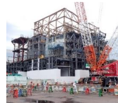
Installing a large cover for Unit 1
