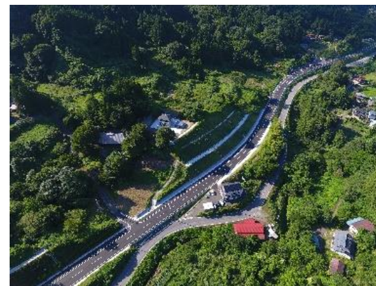
National Route 349 (Otsunagi District in Kawamata Town) In service as of March 21, 2023
