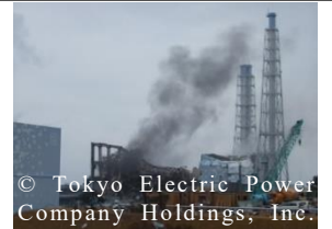
Unit 3 immediately after the hydrogen explosion
