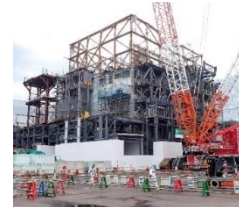
Installing a large cover for Unit 1
