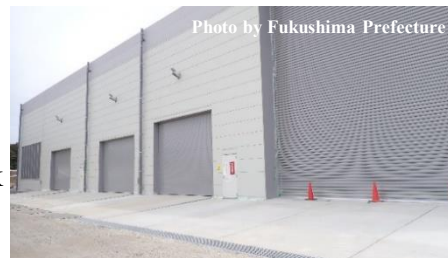
External view of the volume reduction facility
