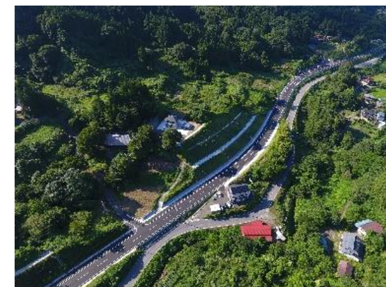
National Route 349 (Otsunagi District in Kawamata Town) In service as of 21 Mar. 2023
