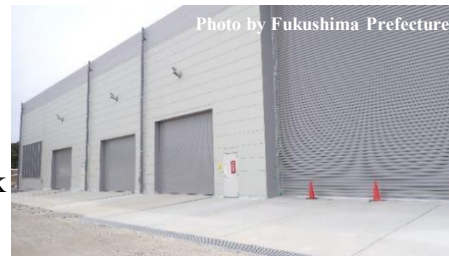
External view of the volume reduction facility
