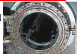
Unit 2 Reactor after removal of deposits from the PCV penetration (©IRID)
