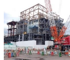
Installing a large cover for Unit 1
