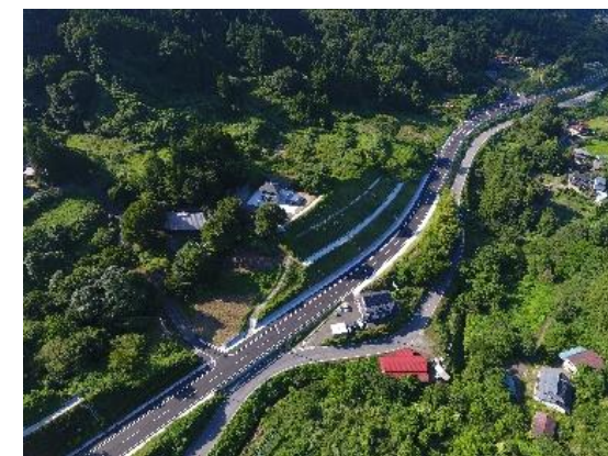
National Route 349 (Otsunagi District in Kawamata Town) In service as of 21 Mar. 2023
