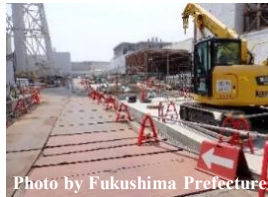
Before facing (near Unit 3)
