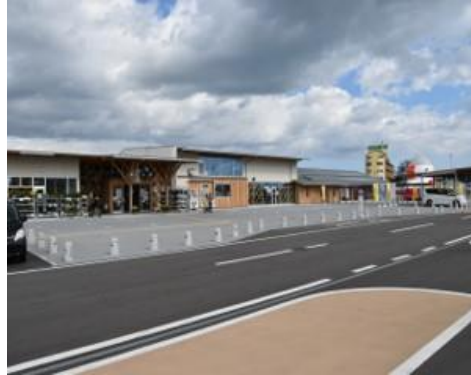
Namie Town: Roadside-Station "Namie"
