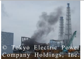
Unit 3 immediately after the hydrogen explosion
