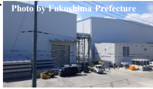
Exterior view of solid waste storage 10 (left: Building B; right: Building A)
