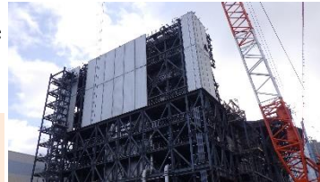
Installing a large cover for Unit 1
