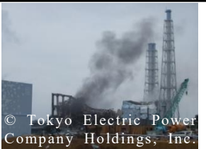
Unit 3 immediately after the hydrogen explosion
