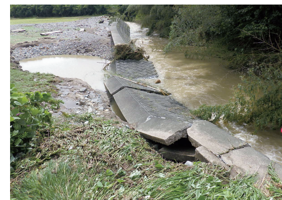
▲ Collapsed embankment at the Fujiwara River (Iwaki City)
