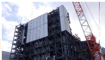
Installing a large cover for Unit 1
