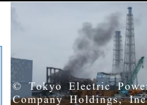
Unit 3 immediately after the hydrogen explosion
