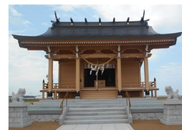
The rebuilt Kusano Shrine
