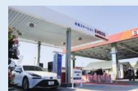
Hydrogen Station in Fukushima City
