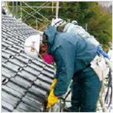
▲ Decontamination of homes (removal of deposited material)
