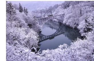
Tadami Line railway facilities
