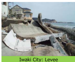
Iwaki City: Levee
