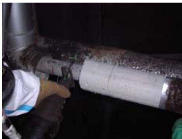
図 4-4-6 配管露出・切断例
